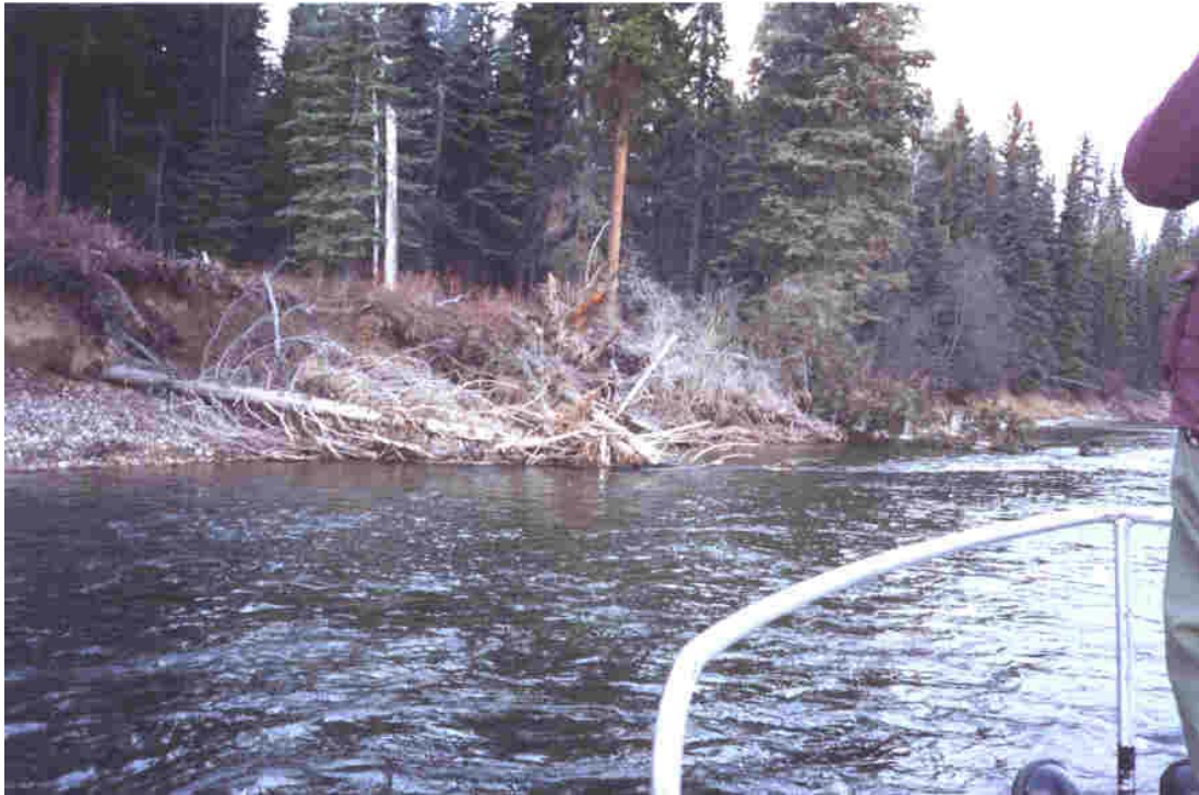
Photograph 7: Downstream boom added to rail anchored sweeper (LM82.1RAS) to improve debris capture (November 1993).
