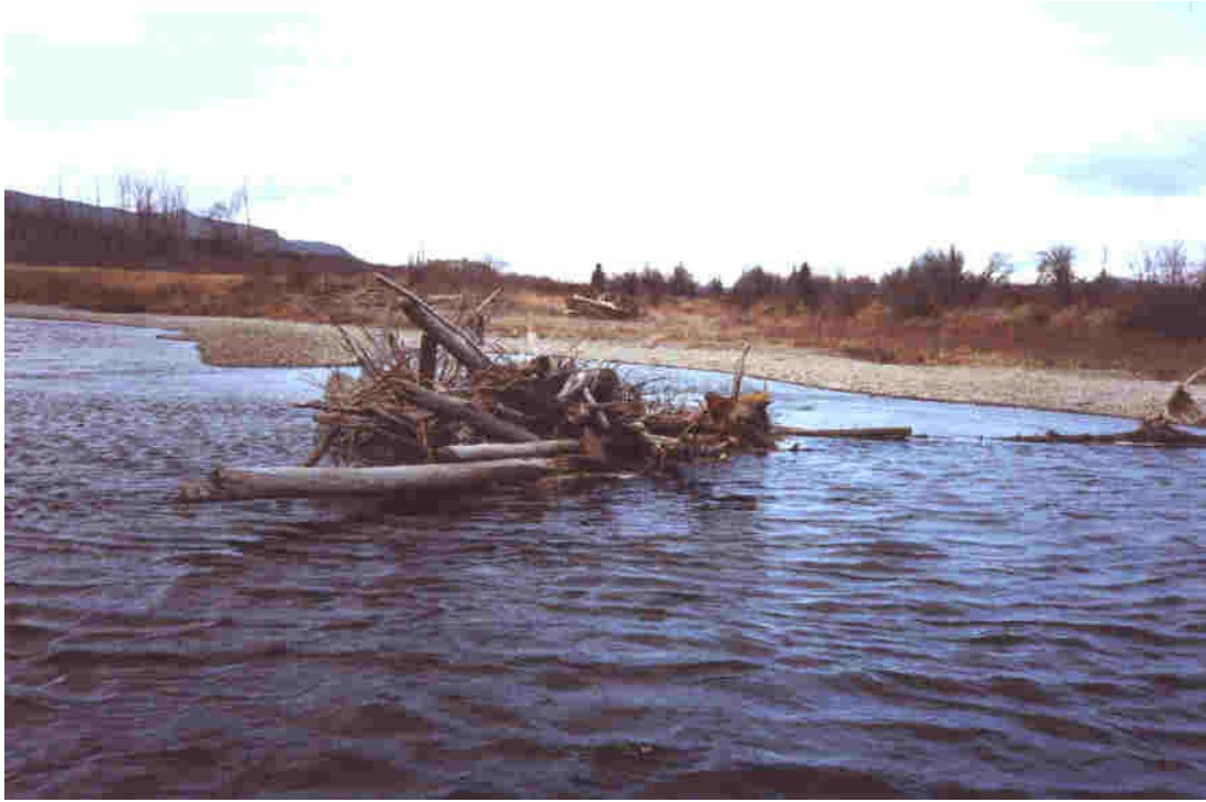
Photograph 13: Rail debris catcher (RM86.375RDC) showing significant debris capture (November 1993).
