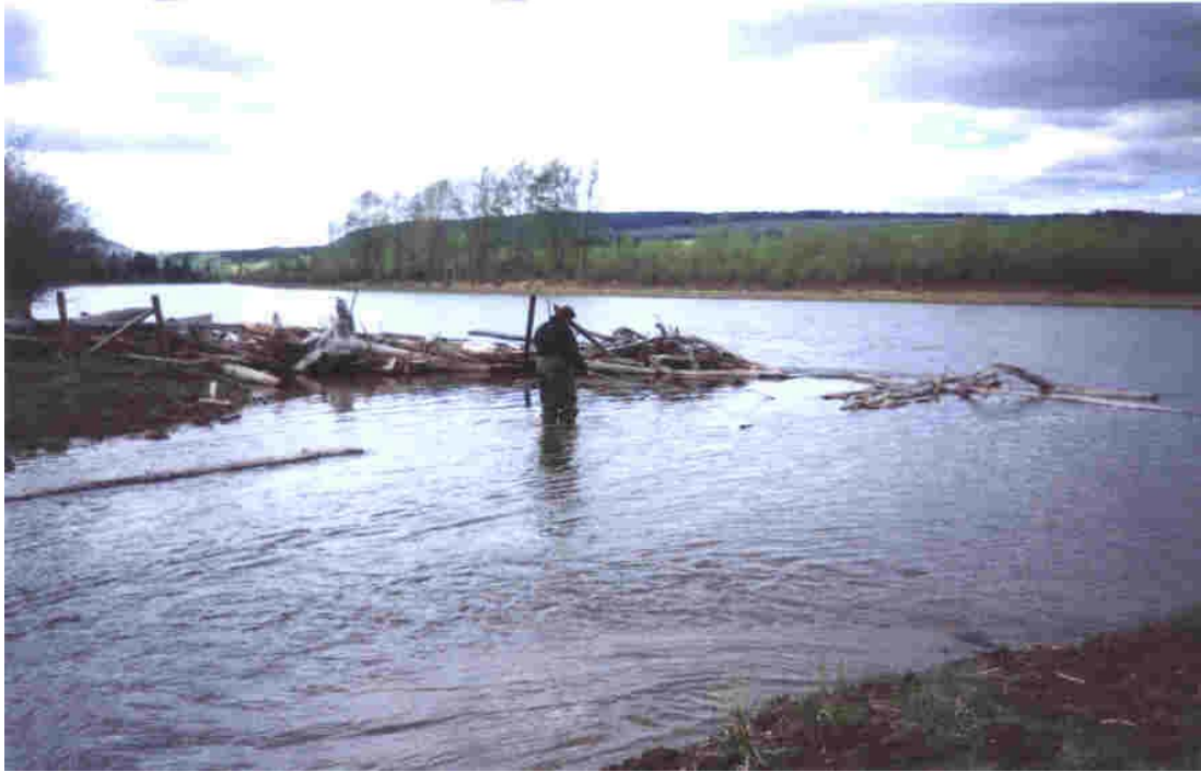
Photograph 11: Smaller pipe-pile debris catcher (RM34.7PDC) providing 42 m 2 of cover area despite loss of downstream pile (May 1995).
