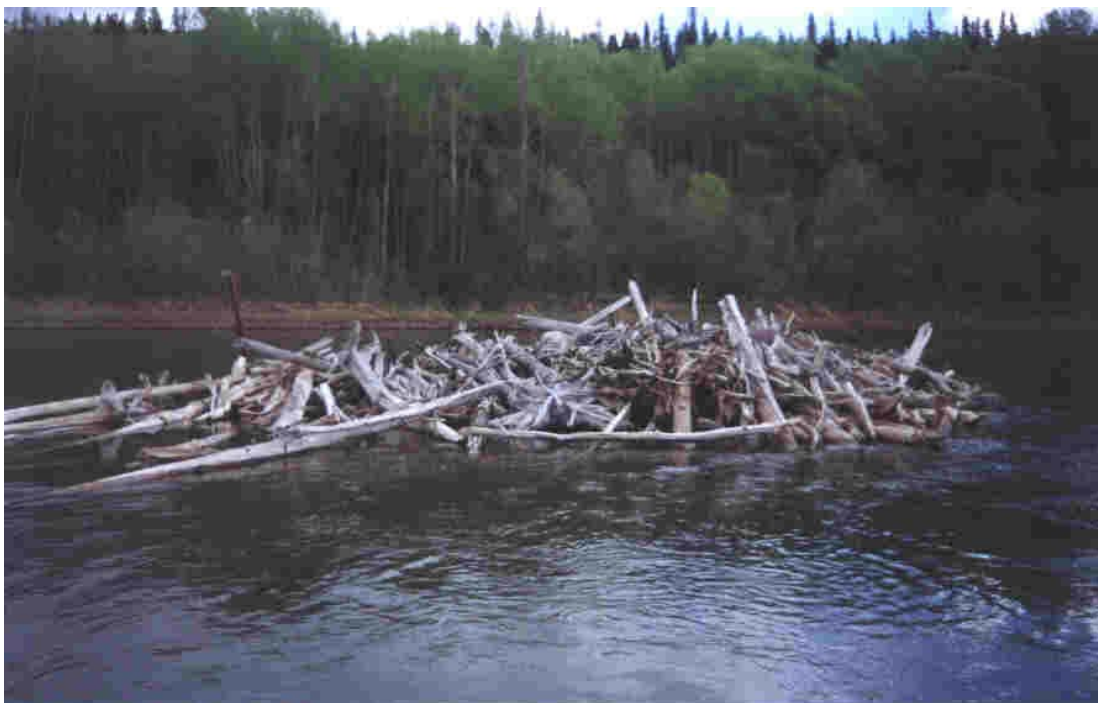
Photograph 12: Large accumulation (149 m 2 ) at pipe-pile debris catcher (MC35.4 PDC, May 1995).
