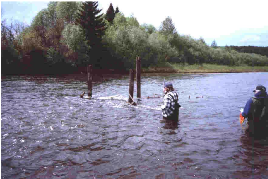
Photograph 14: Rail debris catcher (MC85.6RDC) removed from 1995 physical assessment due to loss of all debris during summer cooling flows (May 1994).
