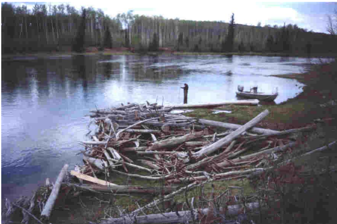
Photograph 4: Floating crib (RM27.4FC) not providing much cover as its upstream end pushed onto the shore (May 1995).
