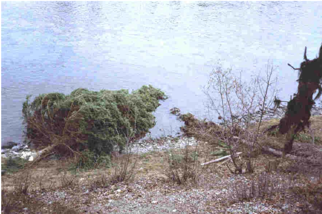
Photograph 9: Downstream boom added to hand-placed anchored sweeper (LM75.9HAS) to improve debris capture (April 1993).
